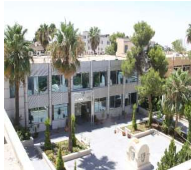
Metal cladding systems
